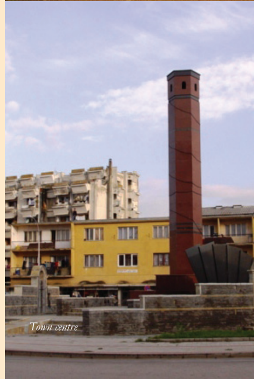
Mark Krustem Jakaj's Tower
